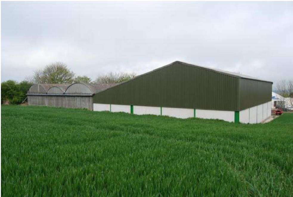
Adjacent buildings view to north west.
