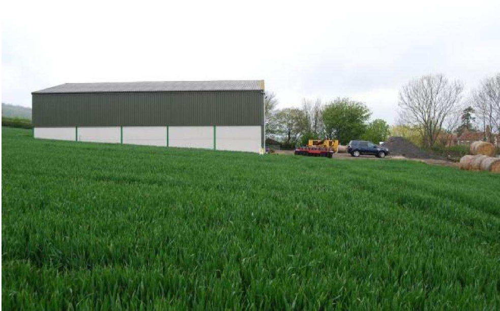
View across site to west.
